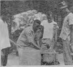
Making Concrete Block
